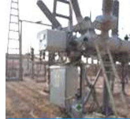
10-Filling with SF6 gas at nominal pressure
