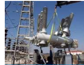
5-Erection of poles Fixing by screws
