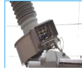
11-Wiring of CT's to local control panel
