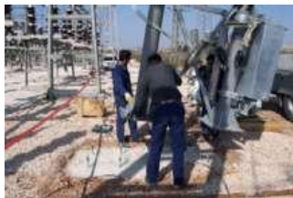
2-Fixing the support by crane
