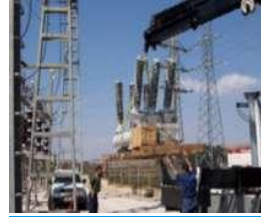
3-Unloading PASS M0 module
