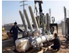
4-Removing the transport structure
