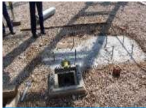
1-Foundation prepared for erection
